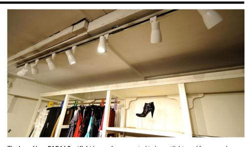
The **Long Nose PAR16 Spotlight** is a surface mounted twin spotlight used for general lighting. It has a longer body than standard GU10 spotlights, meaning that elongated bulbs such as LED retrofit lamps can be used without the light source protruding.
