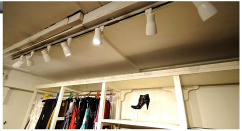
The **Long Nose Track** single circuit track mounted spotlight used in conjunction with our single circuit 240V track ceiling fixtures. It has a longer body than standard GU10 spotlights, meaning that elongated bulbs such as LED retrofit lamps can be used without the light source protruding.
