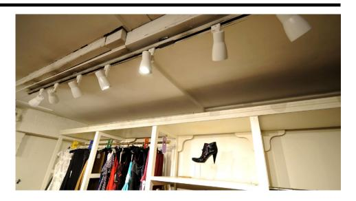
The **Big Nose PAR20** is a surface mounted spotlight with an E27 lampholder, capable of taking PAR20 and R64 reflector lamps with a maximum wattage of 60W.
