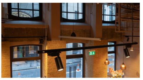
A Three-circuit track lighting is a versatile and flexible lighting system commonly used in commercial and residential spaces and designed to provide maximum flexibility and lighting control in various settings. It consists of a track, which is a metal rail or strip that can hold multiple light fixtures, and each fixture can be independently controlled through one of three separate circuits within the track.
