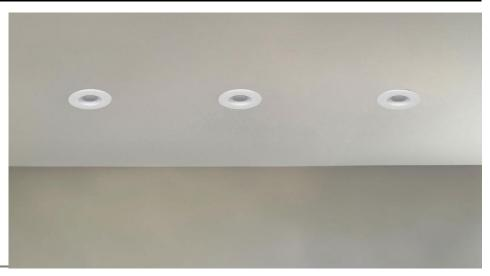
IP65 fire-rated LED downlight with Smart WIFI control, 3000K-6500K tuneable white colour temperature and smooth dimmable operation.
