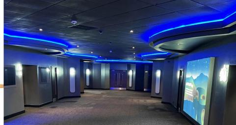
**LED Ropelight 5050** has many benefits over standard ropelight. The advantages include 50,000 hours life, a bright and sharp light source and low power consumption with virtually no heat. This means that it can safely be rebated instead of being surface mounted.
