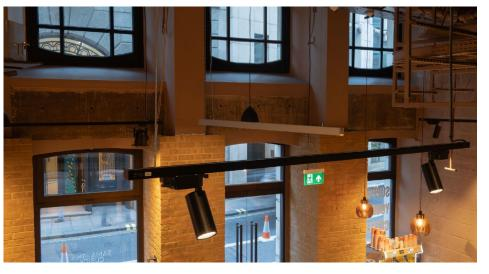
The **Tube Three Circuit Track Lights Range** fittings are 240V dimmable spotlights mainly used to highlight certain focal points. The fittings have a built in LED and a high lumen output, making them low energy and powerful light sources, ideal for commercial or residential use.
