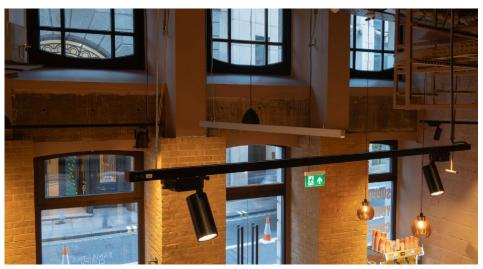
The **Tube Integrated LED Honeycomb Baffle** employs a honeycomb mesh to reduce the glare from the tube light. Commonly used in homes, offices or restaurants where their anti-glare properties can help you concentrate or relax in a gently-lit environment.
