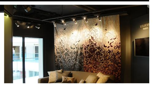
The **PAR30 3 Circuit Theatre Track** lights are 240V spotlights used to highlight certain focal points using different wattages, brightness, beam angles, filters and coloured gels.
