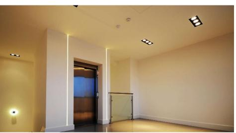
The LED Grid Trimless Triple AR111 is an adjustable downlighter with three 13W AR111 LED Lamps & Drivers.
