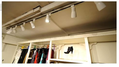
The **Big Nose 100W Three Circuit Track** is an adjustable track fitting spotlight used for general lighting.
