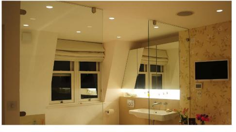
The **Trimless Downlight** is a fully adjustable downlight that is available in round or square, black or white. It is designed to be plastered into ceilings to give a **seamless** appearance. One of the advantages is that the downlight can be installed then plastered and painted.
