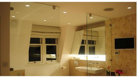
The **Trimless Downlight** is a fully adjustable downlight that is available in round or square, black or white. Using the different lampholders available you can select different light sources; Halogen, LED and Metal Halide. It is designed to be plastered into ceilings to give a **seamless** appearance. One of the advantages is that the downlight can be installed then plastered and painted. Trimless Downlights with LED MR11 Lamp
