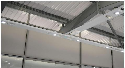
The Multi Suspension LED Emergency Kit is a Multi Suspension Joiner with LED emergency downlight for use with the Multi Suspension Tray System. The Emergency downlight is non-maintained meaning that it only becomes illuminated when there is a power cut; its normal state is off with the 1mm green healthy battery indicator lit. In the event of a power cut the supplied sausage battery pack becomes active and powers the 3 Watt LED for up to 3 hours.
