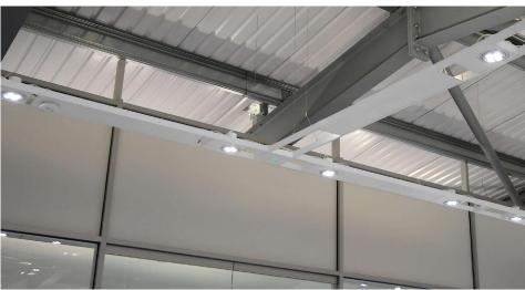
The Multi Suspension Power Suspension Kit is a ceiling base with suspension cable and power cable for the Multi Suspension Tray System.
