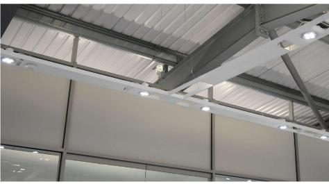
The **CDMT Wall Washer Tray Fitting** is a metal halide fitting for use with the Multi Suspension Tray System.
