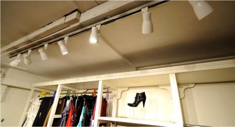
The **Big Nose R80 Spotlight** is a surface mounted spotlight with an E27 lampholder, capable of taking PAR25 and R80 reflector lamps with a maximum wattage 100W.
