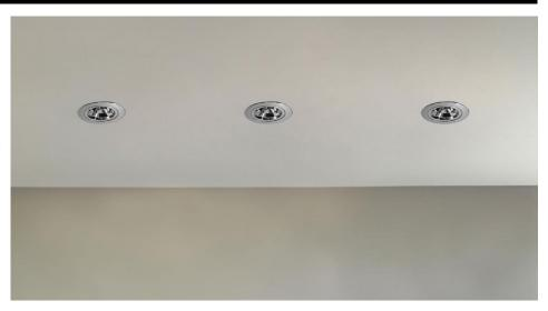
The Long 240V downlight does not require a firehood and is fire rated for up to 90 minutes.
