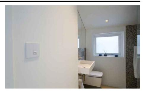
The **Rania Dimming Interface 0-10V** is used with fluorescent and dimmable LED lighting. Fluorescent lighting requires a 0-10V dimmable ballast, LED lighting requires a 0-10V dimmable controller.
